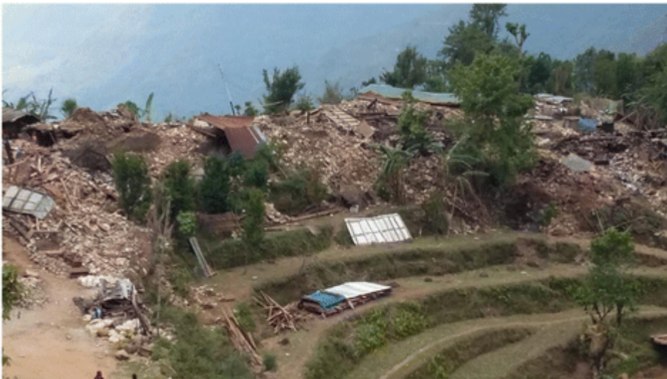
Figure 3: Completely Collapsed dry Stone Masonry Houses
